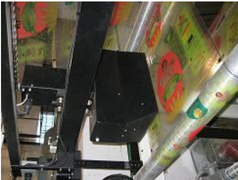
CS4 system installed on Expert Rotogravure Press
